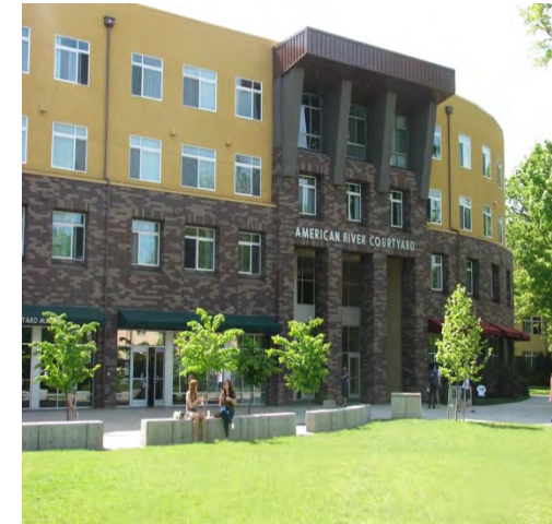
ARC (2009) - 606 Beds Suites & Apartments (limited)
