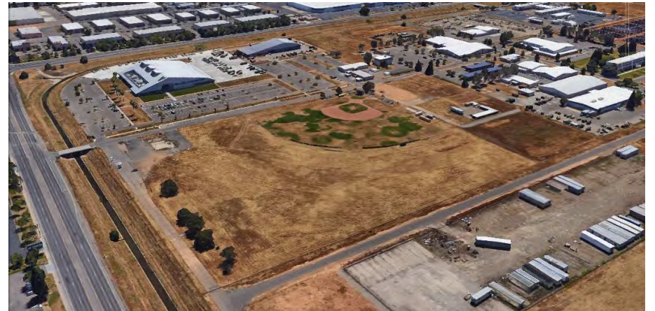
Replacement Ballfields Site
