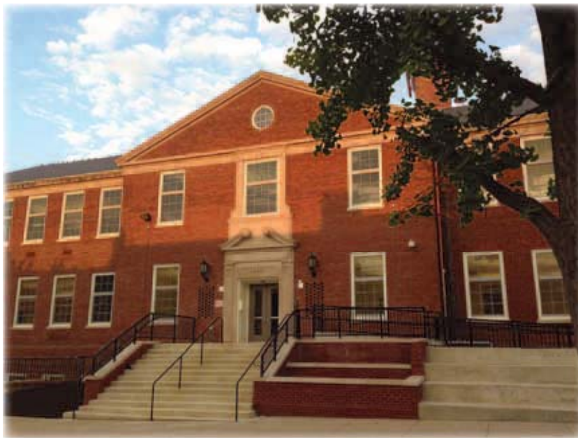
The renovated Randolph building on the first day of school for Washington Latin, September 2013.
