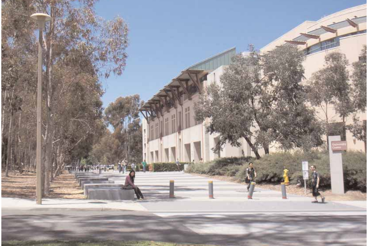
The Center Hall classroom building at the University of California at San Diego is on Library Walk, which forms an edge at University Center, the 24-hour neighborhood emerging at the heart of the campus.
