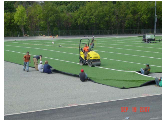
Installation of turf
