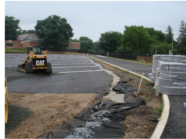
Installation of drainage system
