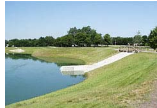
Detention/ Irrigation Basin
